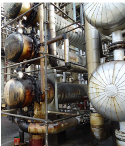
BEFORE: LEAKING HEAT EXCHANGERS
