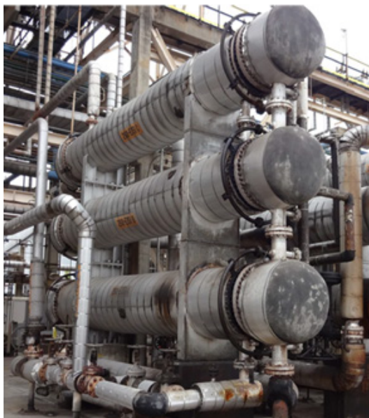
AFTER: LIVE LOADED GASKETS WITH SOLON FLANGE WASHERS
